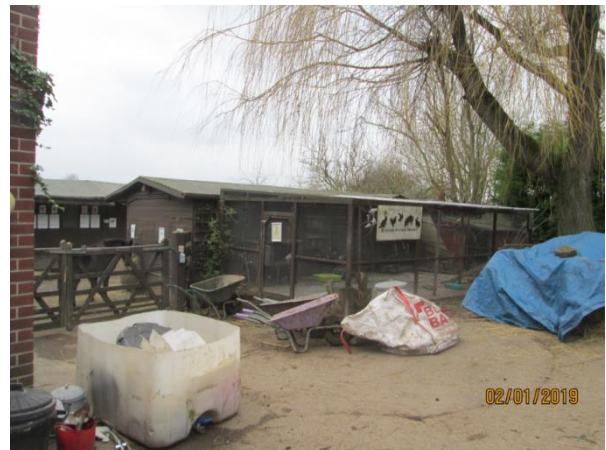
East elevation of existing stable and aviary.
