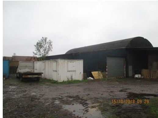
View of main shed
