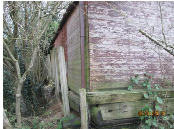
Rear elevation of existing stables.
